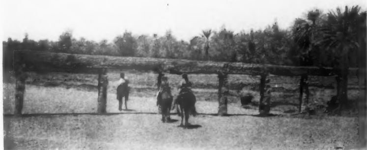
PRIMITIVE AQUEDUCT OF PALM TRUNKS AND MUD, AT MALHAM
