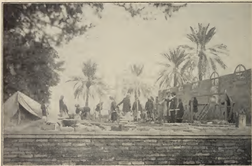
MR. HAYNES SUPERINTENDING THE CONSTRUCTION OF A HOUSE
