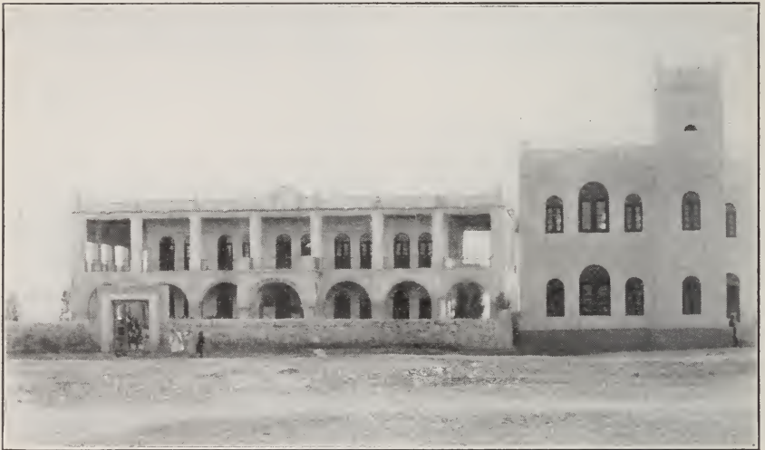
BAHREIN HOSPITAL TO THE LEFT, SCHOOL WITH CHAPEL IN THE SECOND STORY TO THE RIGHT
