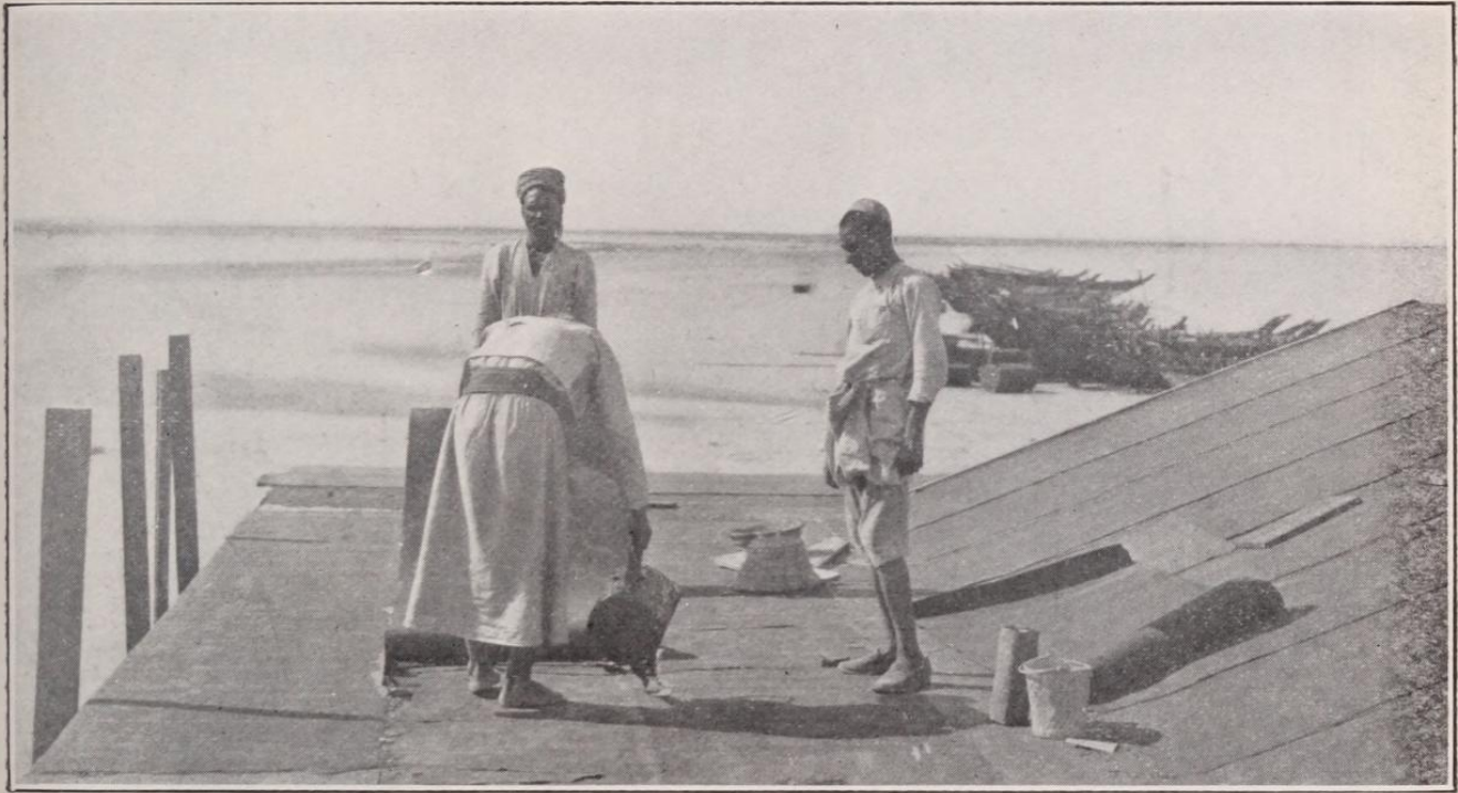
ROOFING THE HOSPITAL.
