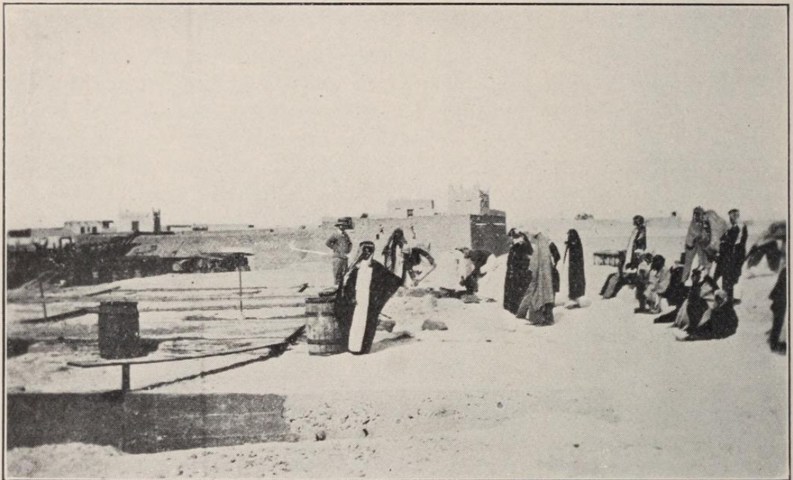
BEGINNING WORK ON MISSION HOSPITAL AT KUWEIT. MR. SHAW SUPERINTENDING
