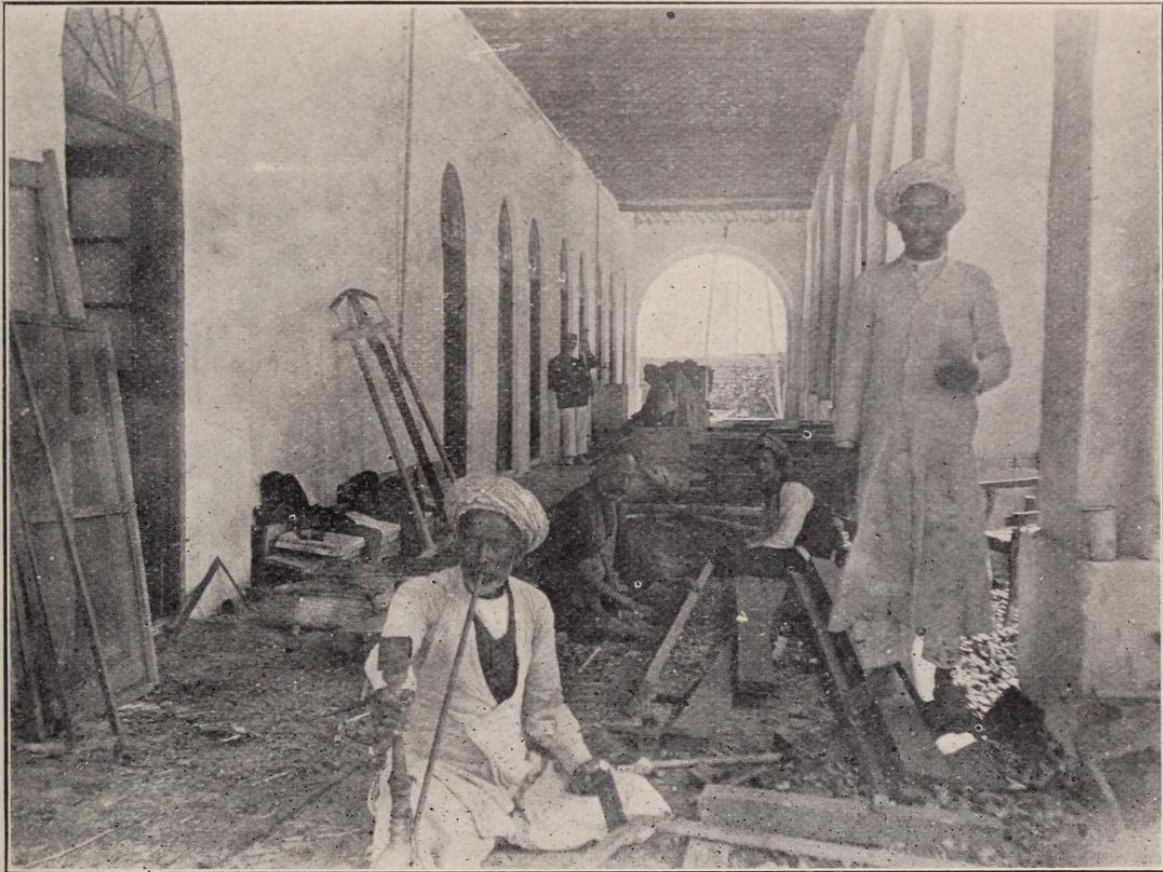
THE CARPENTER SHOP ON THE HOSPITAL VERANDAH AT BAHREIN. These men have made all the doors and windows for the Mission in this place.
