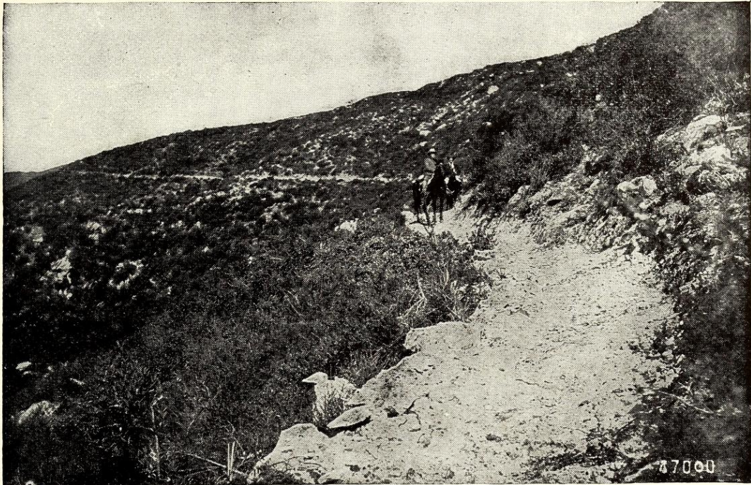
A MOUNTAIN TRAIL, BUILT FOR FIRE PATROL
